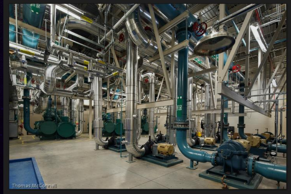
TACC Machine Room Chilled Water Plant
